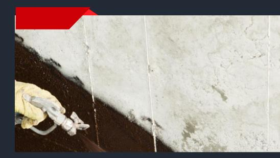
Liquid Armour<sup>®</sup> is available in a Spray form. This allows you to vary the thickness to meet the full range of threat and weight criteria.
